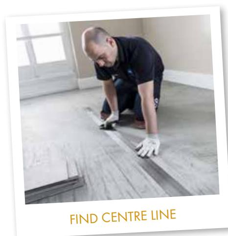
3. Dry lay one plank per row (without adhesive) from this centre line to the wall and ensure no small cuts are needed. Take away these planks.
